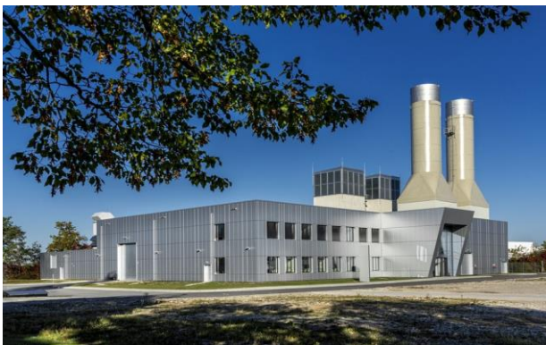
Fig. 1: Airbus Test Center for integrated propulsion systems
